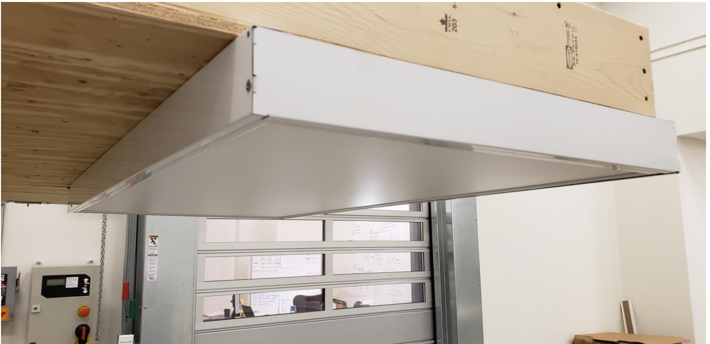
5. Push fixture all the way in and fasten the remaining end cap.
