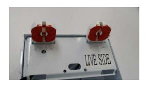
5- Install red sockets to one end of the fixture.
