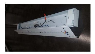
5 - Place 4RB or 8RB LED board and wired driver wirecover on appropriate existing 4' or 8' channel
