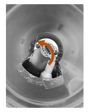
The swivel head is used to center the male G24q socket extender in the fixture.
