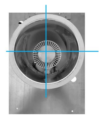
The Lunera CFL LED G24q Type B lamp has been installed in a single or dual horizontal socket fixture that has been connected to line voltage and with the lamp now oriented down, but yet centered in the fixture.
