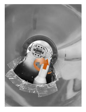
The articulated extension arm is used to extend and rotate the male G24q socket to future center it in the fixture.
