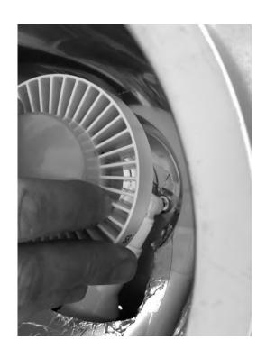
Insert the extended CFL LED G24q Type B lamp into the fixture's G24q socket.
