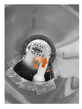
The articulated extension arm is used to extend and rotate the male G24q socket to future center it in the fixture.
