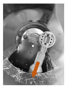
The socket adaptor accessory is installed in one of two G24q horizontal socket, which would result in an offcenter lamp installation.
