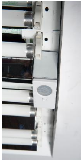
Close-up of Integral Occupancy Sensor in 6 Light Only
