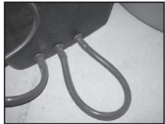
Unused outlets connected with tubing
