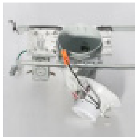
STEP 3: Insert male connector into female one.
