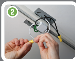
Connect track to mounting plate and wire.
