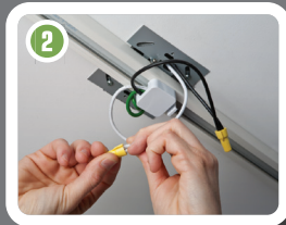
Connect track to mounting plate and wire.
