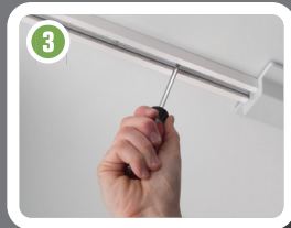
Attach track to ceiling.
