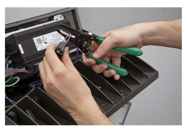
6) Route the new wires through the wire way hole in the housing.
