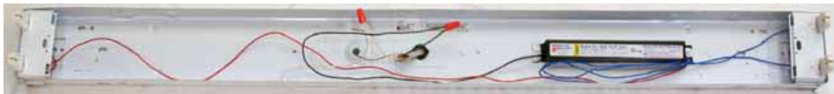
BEFORE (WITH BALLAST AND ORIGINAL LAMPHOLDERS)
