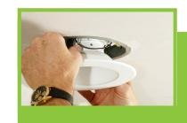
**4**. Squeeze torsion springs and insert into housing receivers. Push DLR56 flush with ceiling.
