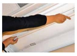
3. Cut the wire connected to the ballast.
