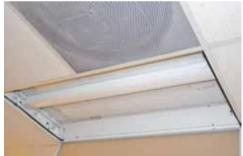
8. Put the new LED tube to the fixture and power on for testing.
