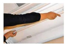
3. Cut the wire connected to the ballast.
