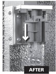
**NOTE:** These lamps have a quartz jacket. Fingerprints and oils must be wiped off prior to operation.
