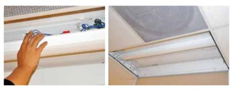
8. Put the new LED tube to the fixture and power on for testing.
